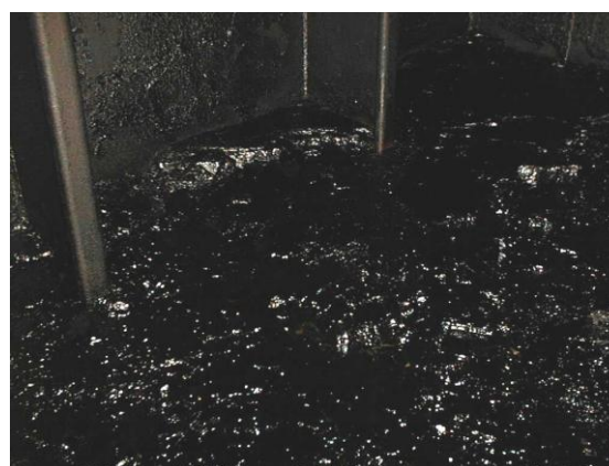
Fuel tank sludge caused by mixing incompatible fuels
